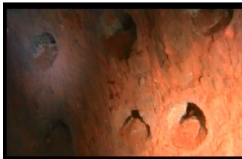
Pic 1. Filter porous clogged by salt and metal corrosion products
