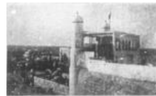
View from the top of Arch
