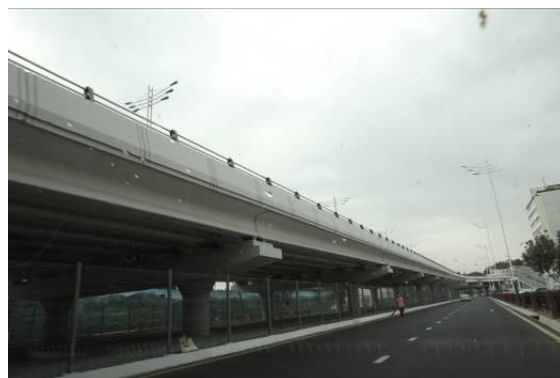
Bridge on the streets Mukimi and U.Nosir
